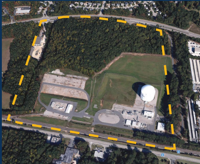
PSNC Energy Utility Site as it exists today.
