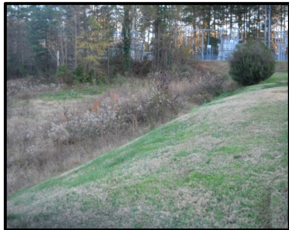
Drainage ditch looking upstream
