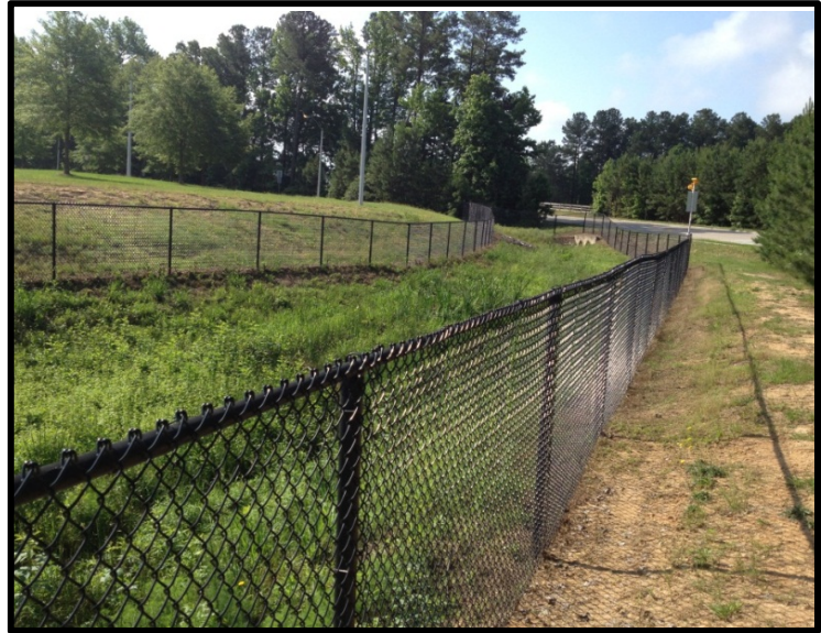
Existing dry detention basin serving Green Hope Elementary
