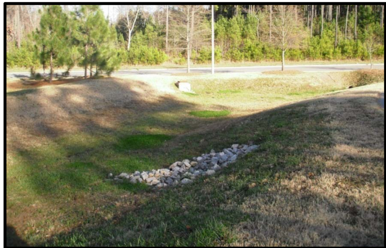
Existing dry detention pond
