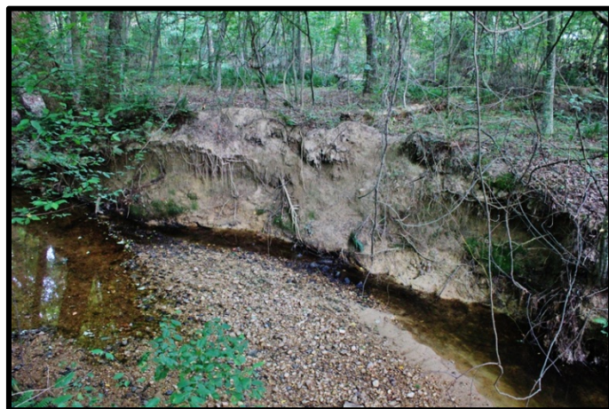
Eroded stream bank by White Oak Creek Greenway
