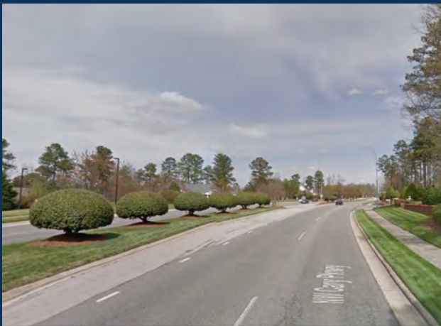
The section of Cary Parkway shown to the left provides a very finished, manicured landscape suitable to suburban development. Note the regular spacing of ornamental shrubs in the median, linear concrete sidewalk, and neat lawn areas.
