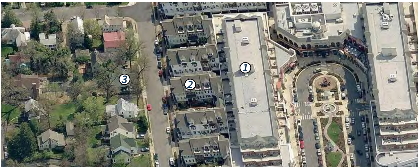
Arlington, VA: Aerial View of Architectural Transitions
