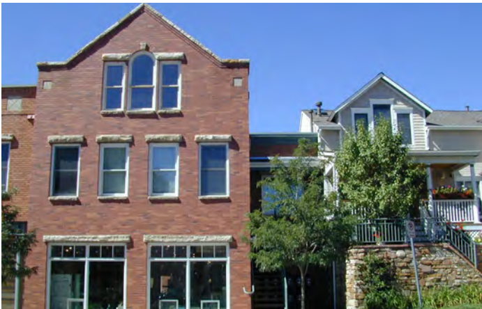
ARCHITECTURE: Boulder, CO
