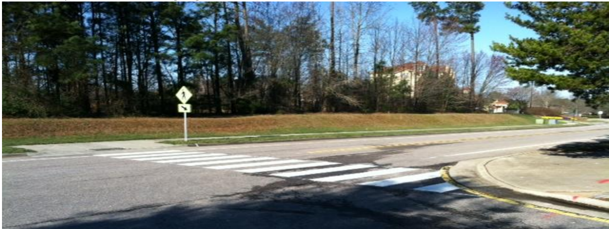
New Safety Crosswalk and Signage on Crescent Commons Drive (Route 5)
