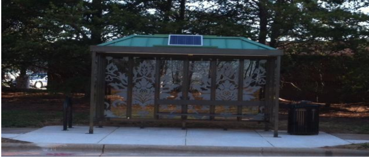
New Passenger Shelter on Crescent Commons Drive (Route 5)
