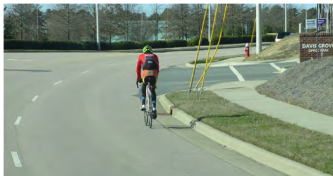
Wide outside lanes on Davis Drive
