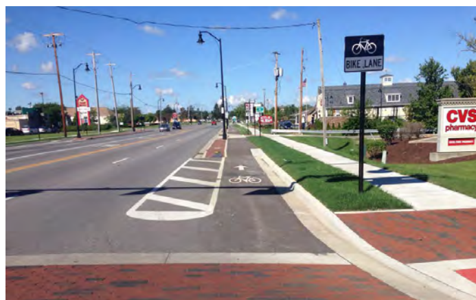
Separated bike lanes with a raised median as vertical separation (Not currently in use in Cary)
