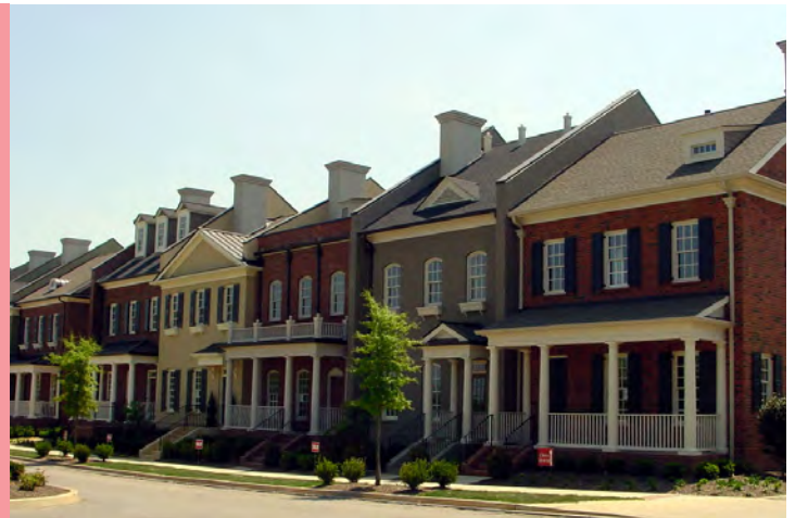
Attached housing with consistent setbacks and varied facades
