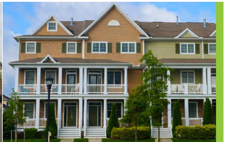
Attached single family and multifamily housing
