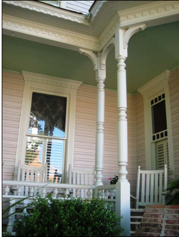
Front porch detail
