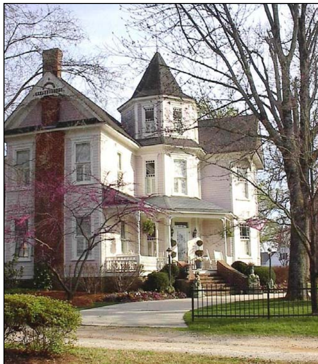
Façade (northwest corner)
