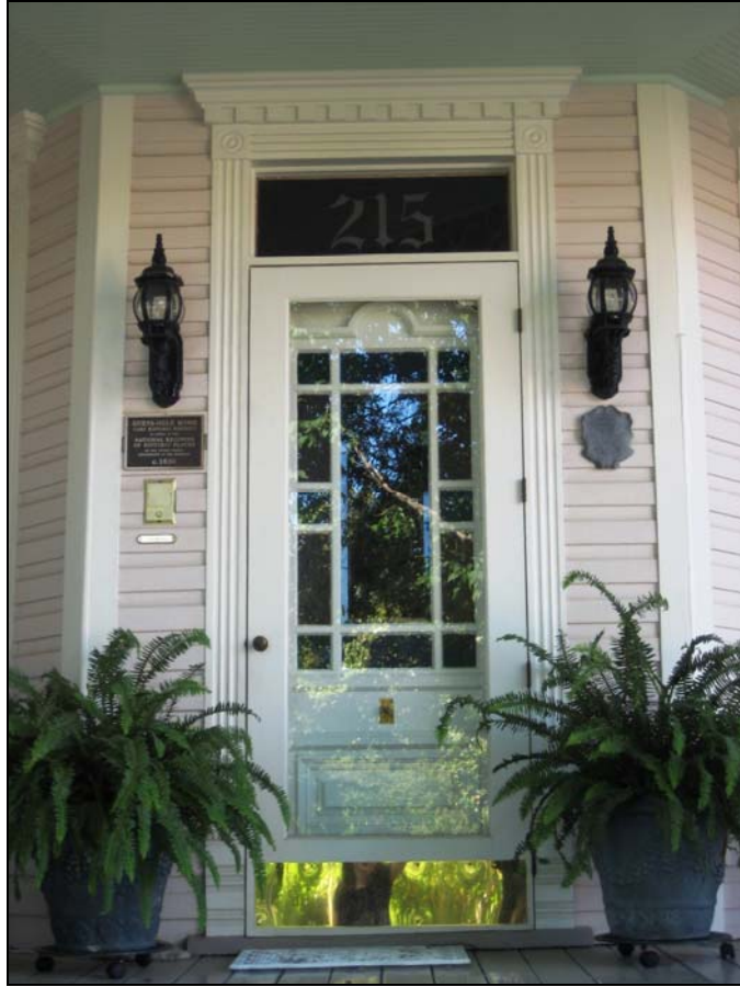
Front entrance detail
