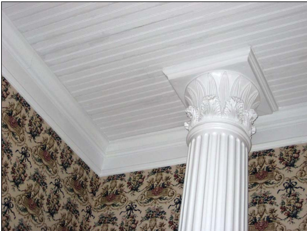
Interior column detail (in foyer)
