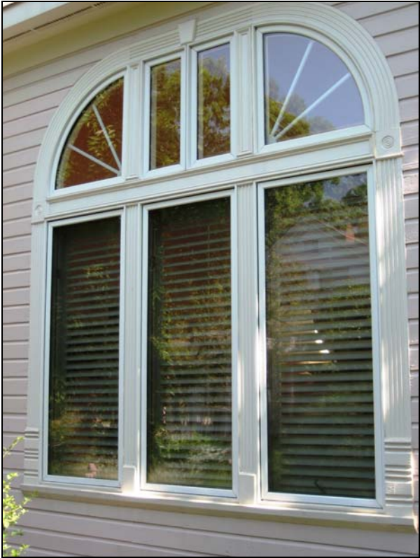
Window detail (on addition, late 1990s, southeast corner)
