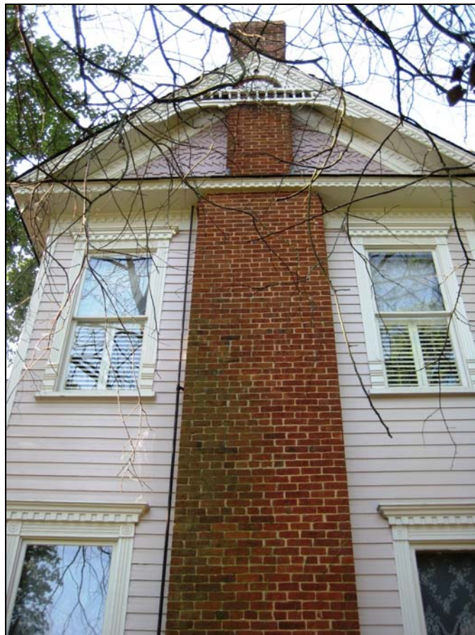
Chimney detail from north elevation
