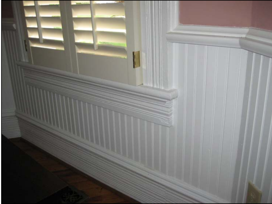
Wainscot and baseboard detail
