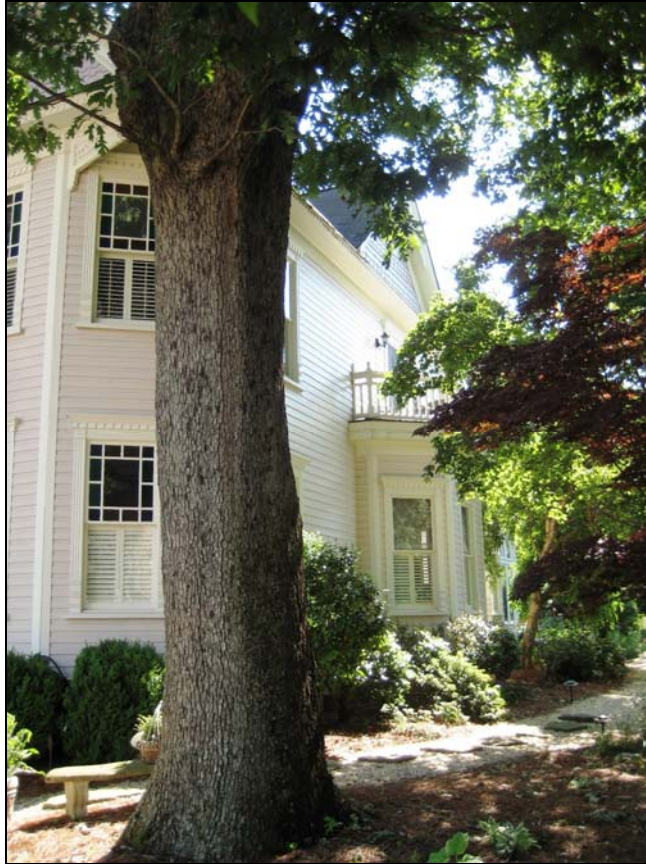
View of South Elevation from southwest corner
