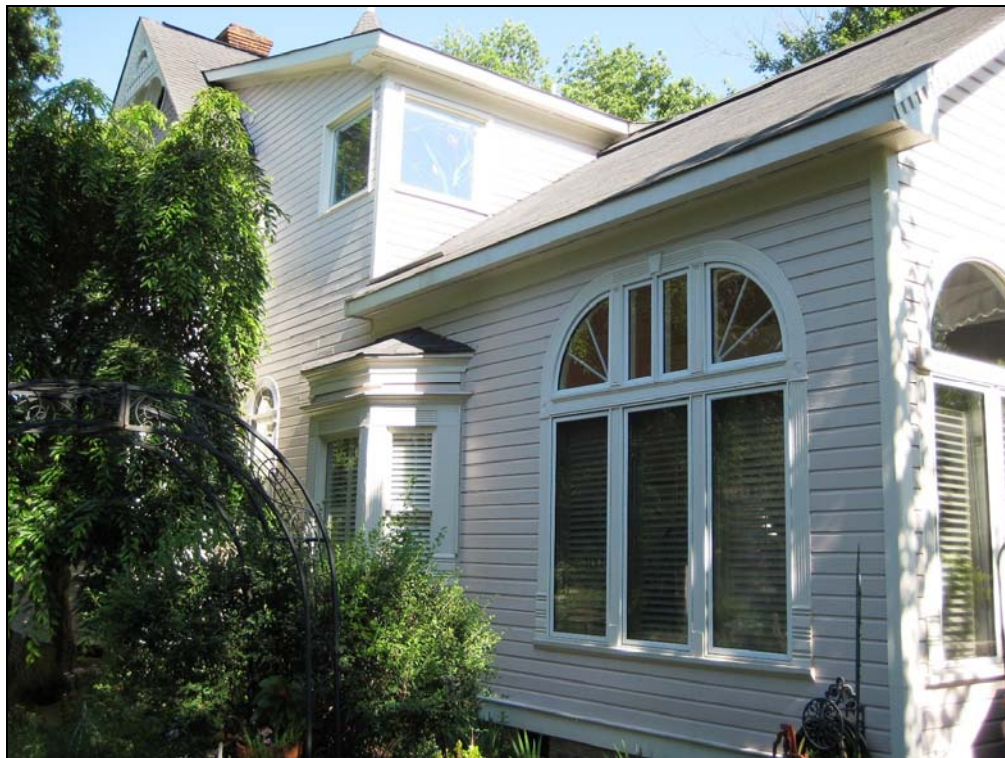
View of South Elevation from southeast corner
