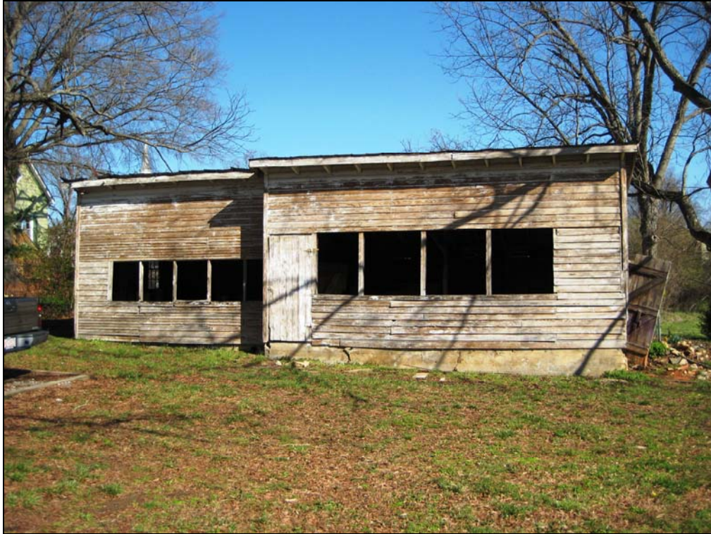
Chicken Coop (façade – south elevation)
