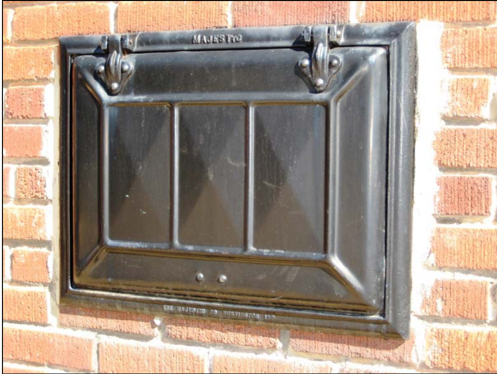
Furnace Hatch (South Elevation)
