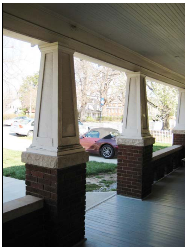
Front Porch (detail)
