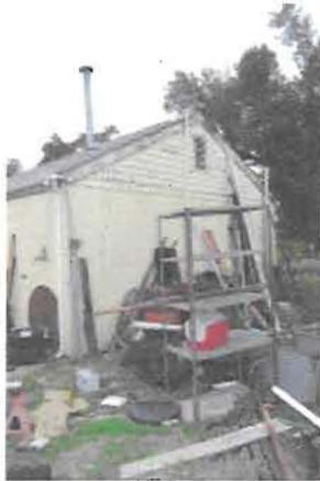
LM_CarpenterFarmSupplyCompanyComplex_store's rear garage addition rear elevation.JPG
