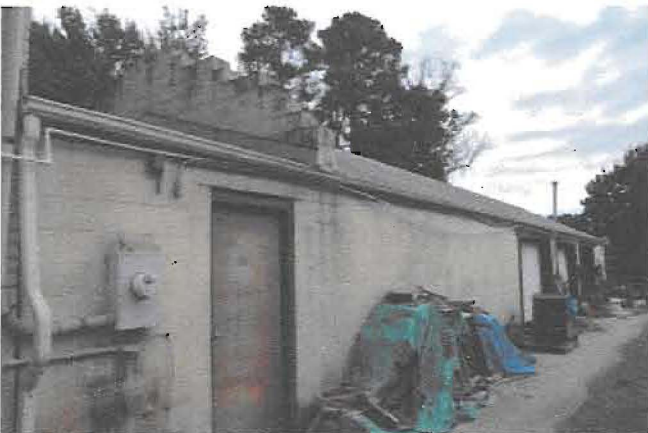
LM_CarpenterFarmSupplyCompanyComplex_store's rear garage addition south elevation.JPG
