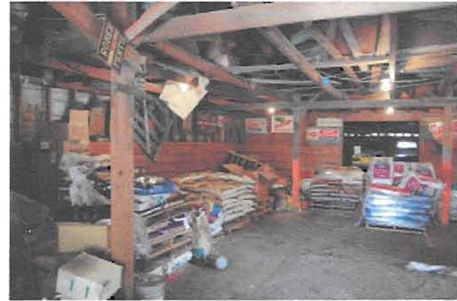
LM_CarpenterFarmSupplyCompanyComplex_co-op addition interior.jpg
