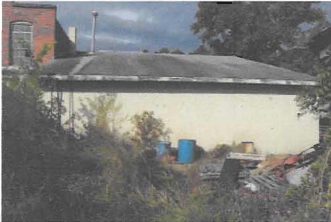
LM_CarpenterFarmSupplyCompanyComplex_store rear elevation.jpg
