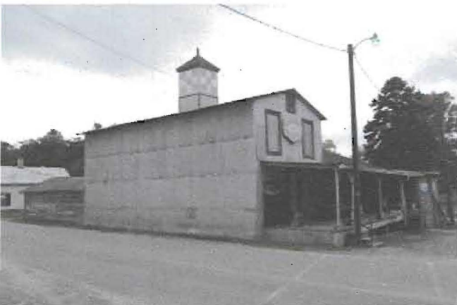
LM_CarpenterFarmSupplyCompanyComplex_co-op east elevation.jpg
