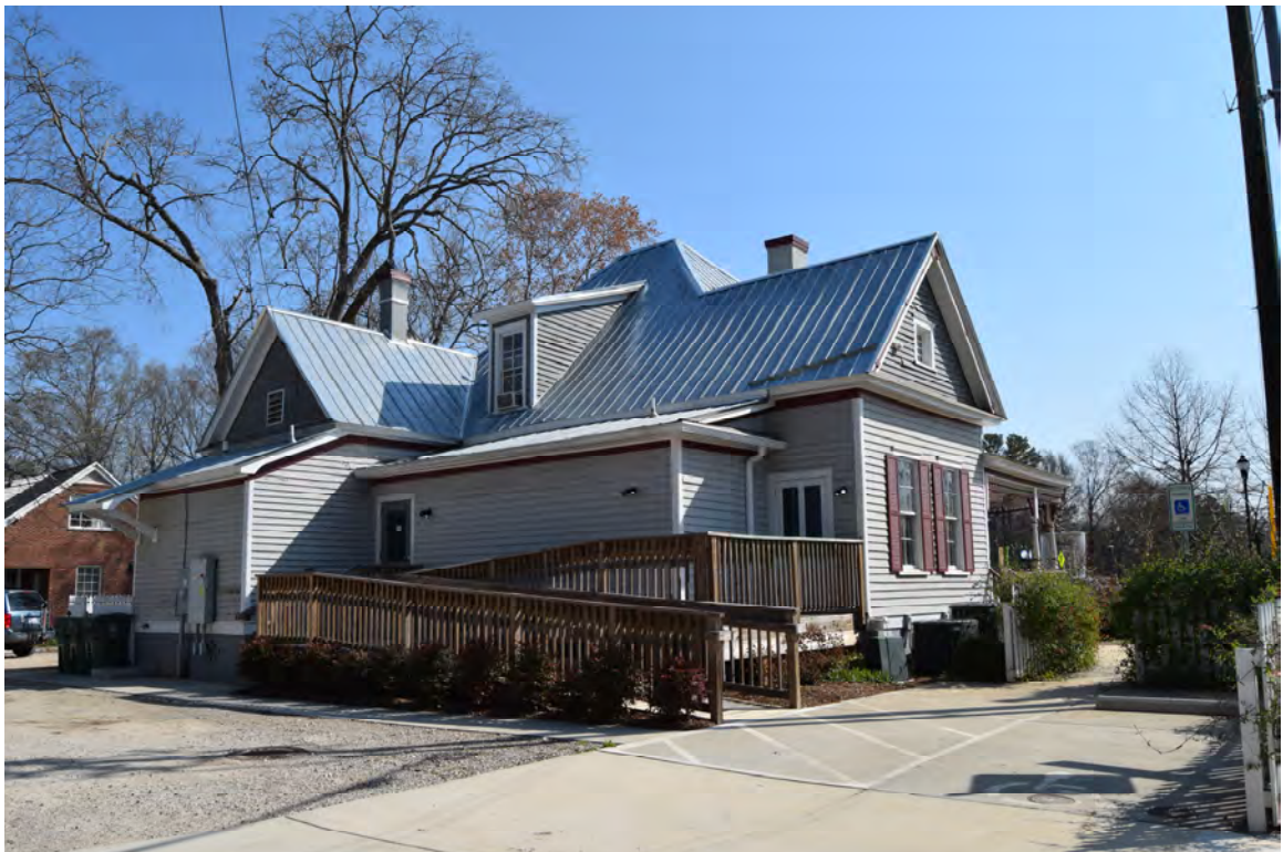
Rear elevation, Sams-Jones House, 324 S. Academy Street, Cary
