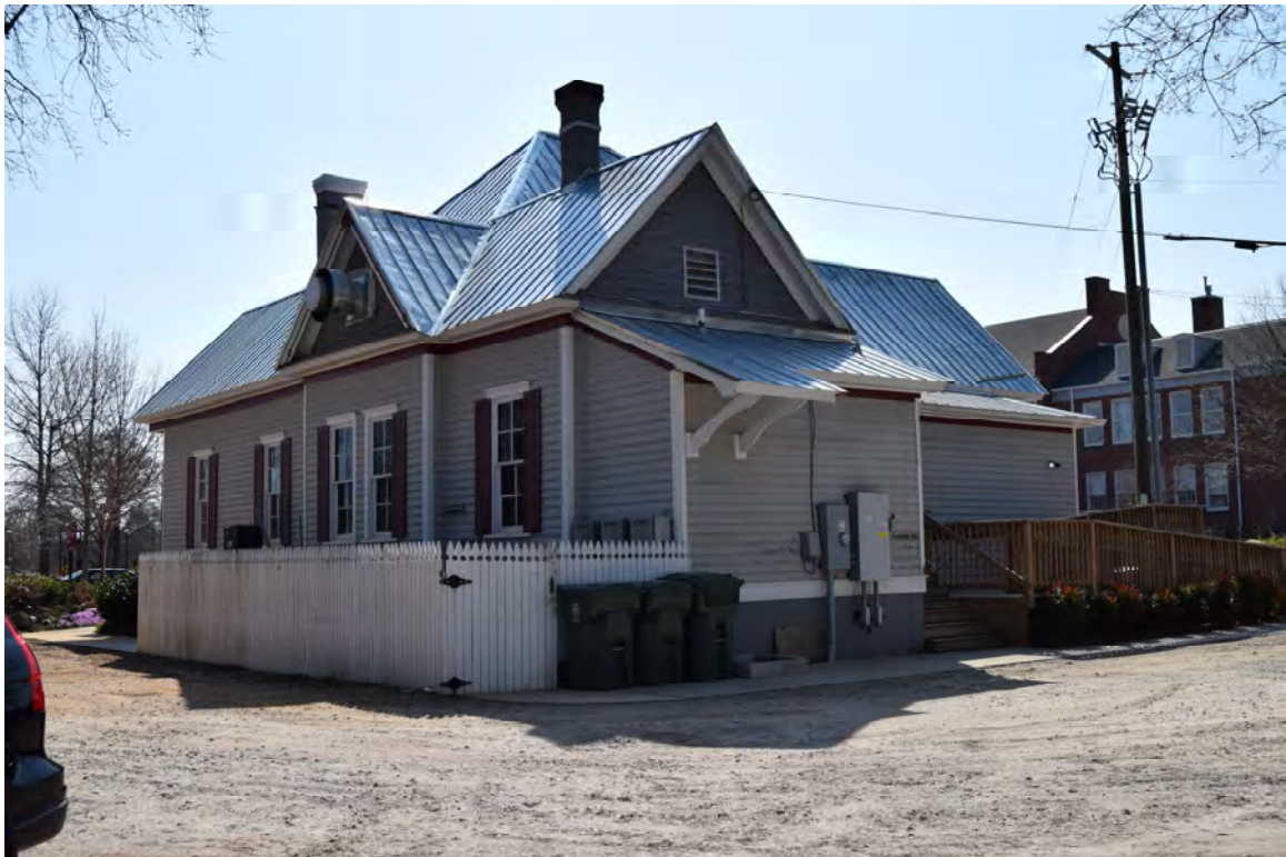
Rear and North elevations, Sams-Jones House, 324 S. Academy Street, Cary
