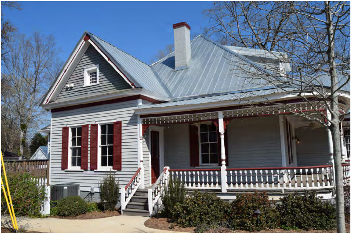
South elevation, Sams-Jones House, 324 S. Academy Street, Cary
