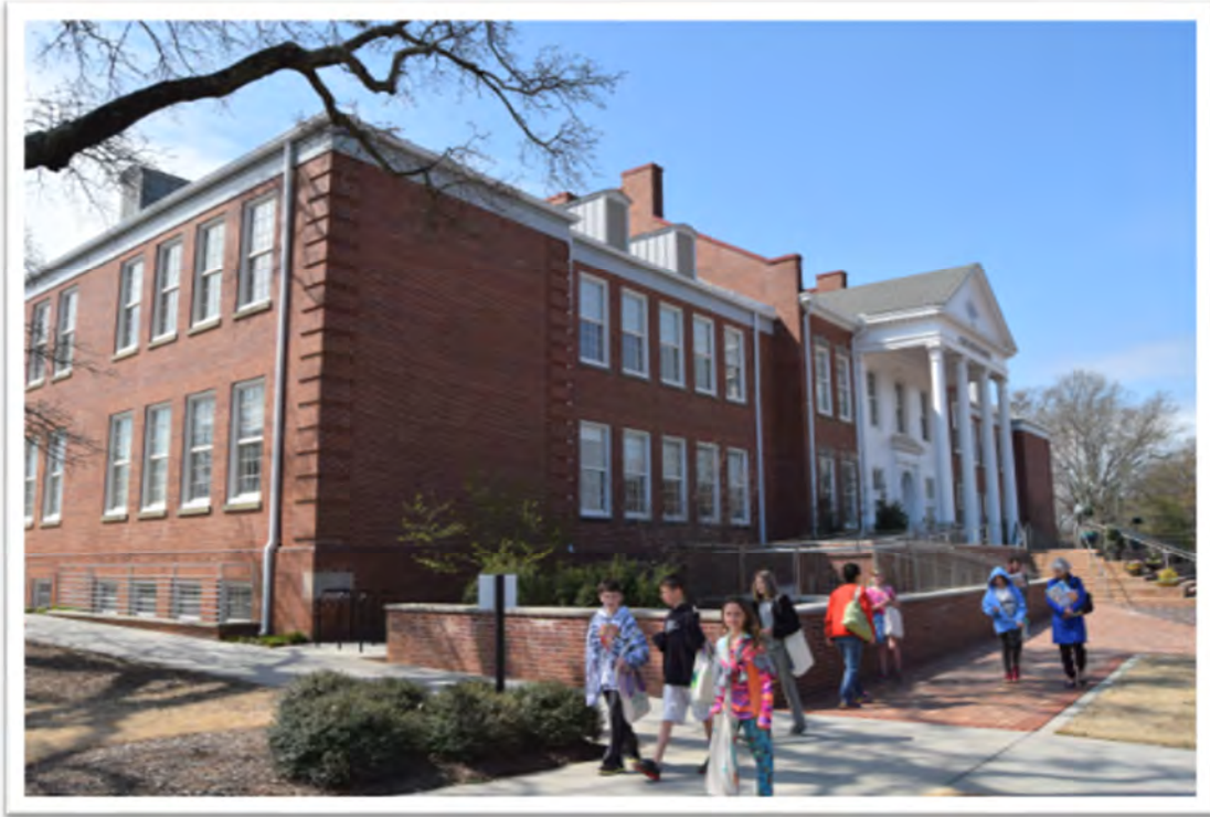
Cary High School, NE corner
