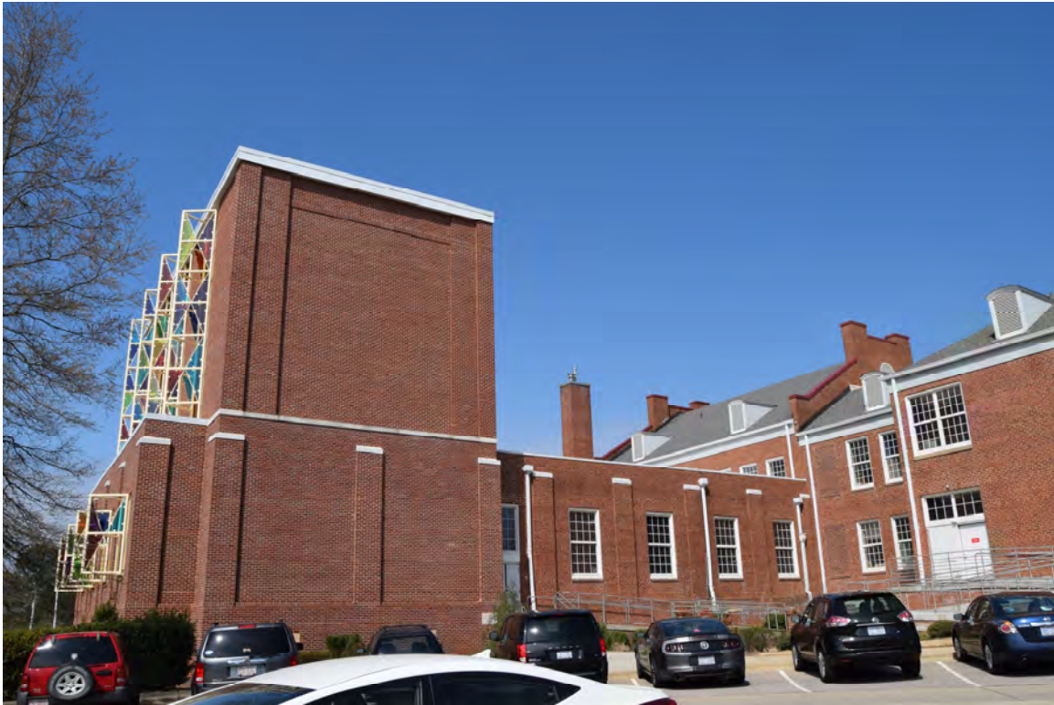
Cary High School, E elevation, auditorium wing
