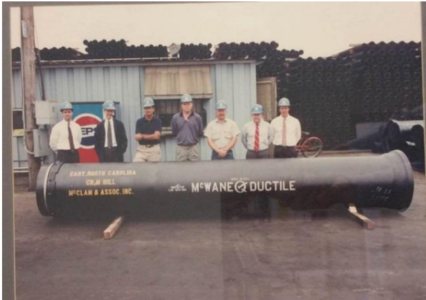
DELIVERY OF THE FIRST PIPE FOR THE CARY-APEX WATER TREATMENT FACILITY RAW WATER PIPELINE, EARLY 1990S
