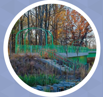
Rock Creek Trail Pedestrian Bridge 2003-2011, Silver Spring, MD Vicki Scuri SiteWorks with URS and Montgomery County Parks & Planning Sponsored by Montgomery County Department of Parks & Planning and Public Art Trust
