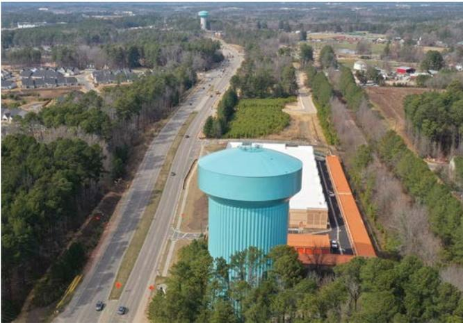
Rehabilitation of the two-million-gallon Carpenter elevated water storage tank is substantially complete. The exterior and interior of the 20-year-old tank received fresh coats of paint with a new perimeter fence and entry gate added on the property. The interior of the tank will be cleaned, disinfected, and placed back into service in early spring, ready to serve the citizens of Cary and maintain reliable water service for another 20 years.
