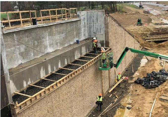
Work is complete on the textured architectural concrete walls for the bridge overpass that supports the CSX railroad over Carpenter Fire Station Road. The textured walls are reminiscent of the architectural features located within and adjacent to the Carpenter Historic District. Work on this project is 65% complete. In February, staff hosted a public listening meeting to share project progress and seek feedback on the project's potential roadway connections, street closures, and street renaming.
