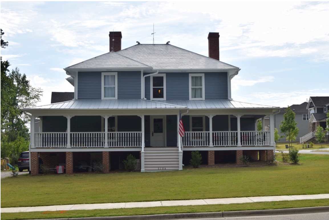
John L. and Henrie G. Sears House, façade, view E
