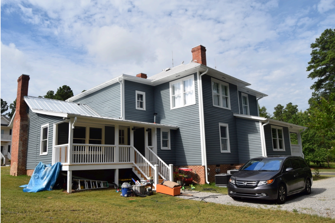
John L. and Henrie G. Sears House, N elevation, view SW
