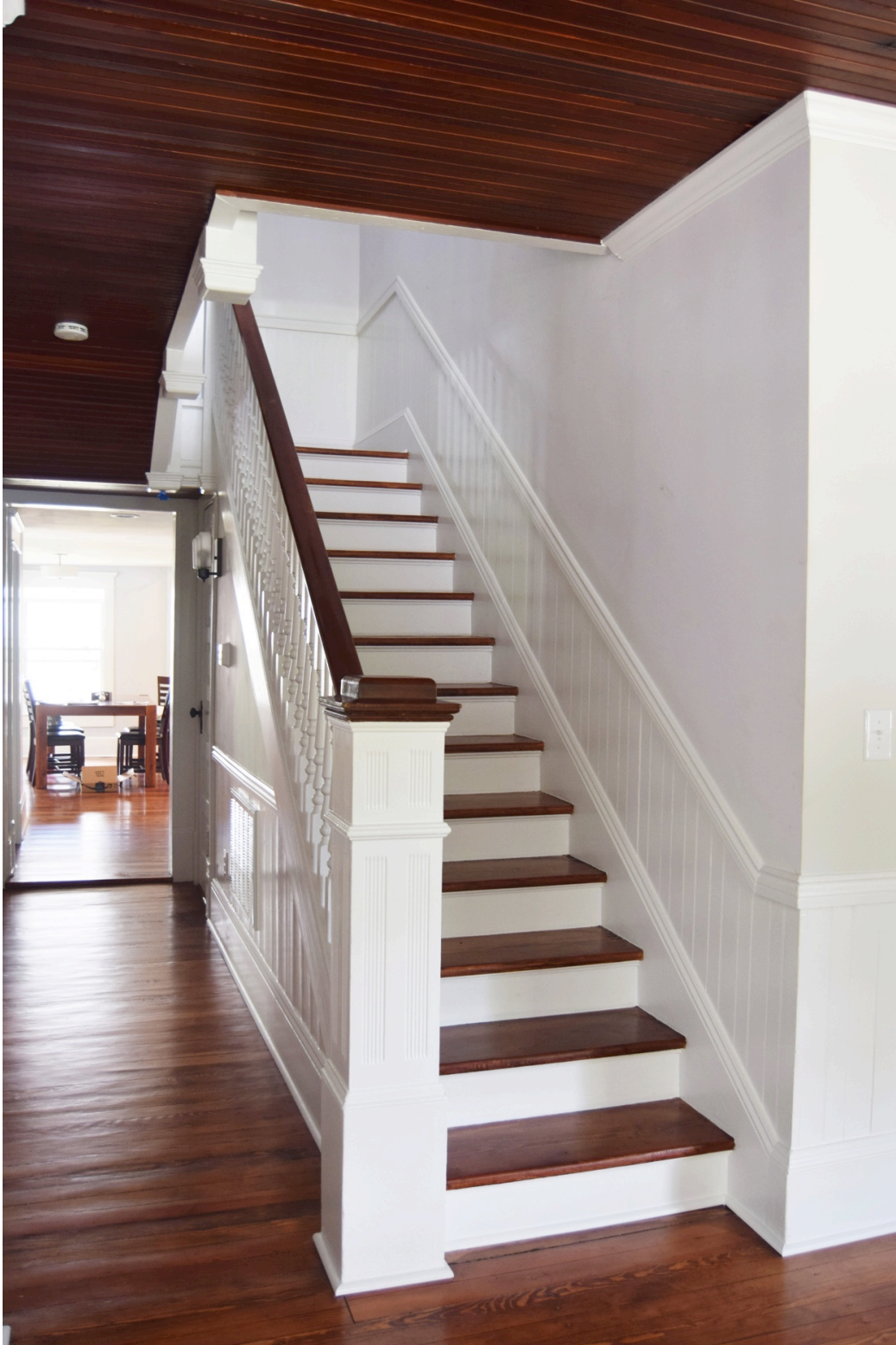
John L. and Henrie G. Sears House, stair hall showing reeded stair newel, view NE
