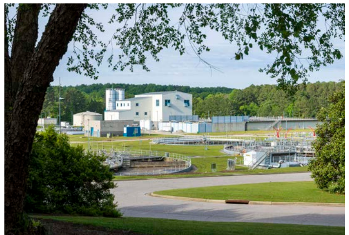
Reclaimed water is a valuable resource produced from wastewater that is highly treated using not only a biological nutrient removal and filtration process, but disinfection with ultra-violet light and Sodium Hypochlorite. The State of North Carolina permits Cary to divert a total of about five million gallons per day from our two treatment plants water reclamation facilities for reuse rather than discharging into creeks.
