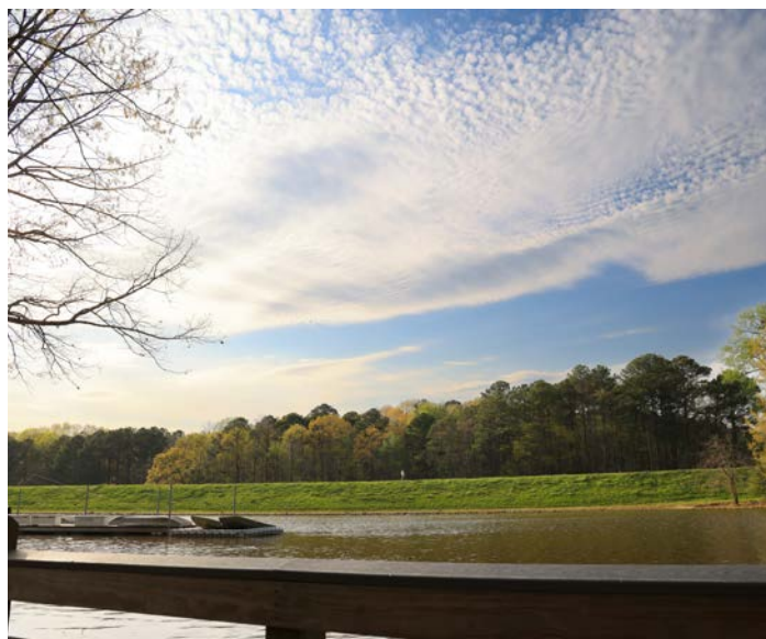
Bond Lake, located within Cary’s Fred G. Bond Metro Park, was constructed by Wake County and the U.S. Department of Agriculture in 1972 as a flood-control structure, and is maintained by Wake County.
