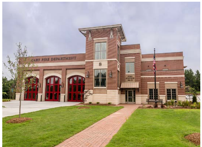
Cary Fire Station 8, on Mills Park Drive, implemented Leadership in Energy and Environmental Design (LEED) principles. These include the use of high-efficiency equipment to reduce energy usage, using the Town's reclaimed water line to reduce water usage, and bicycle storage. Fire Station 8 is also the office for one of the Police Department's GeoPolicing districts.
