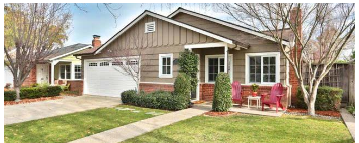
A Strong Neighborhoods Initiative (SNI) was established by the City of San José, California, and partner organizations to strengthen the city's neighborhoods by building clean, safe and strong neighborhoods with independent, capable, and sustainable neighborhood organizations. By coordinating and combining resources, the Initiative is helping neighborhoods reach their full potential as highly livable communities.
