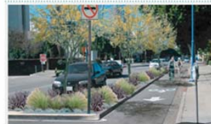
This photo simulation, from Long Beach CA, shows how curbs and landscaped medians can separate bike lanes from through traffic.
