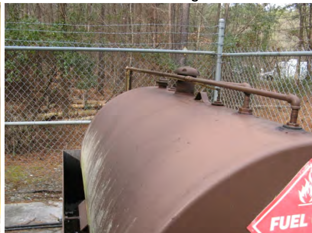
Generator Fuel Tank 600gal
