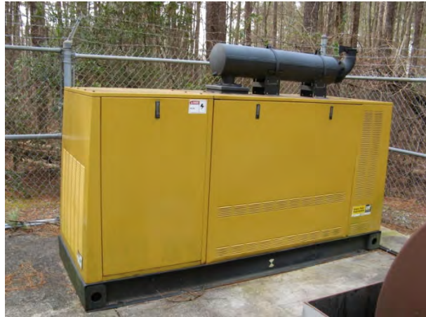
Generator Fuel Tank 600gal
