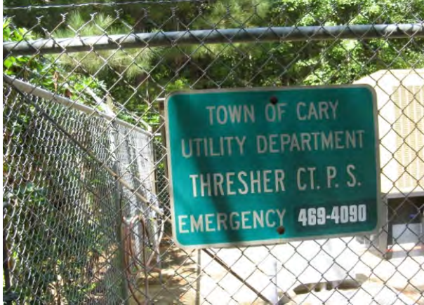
Thresher Court Pump Station
