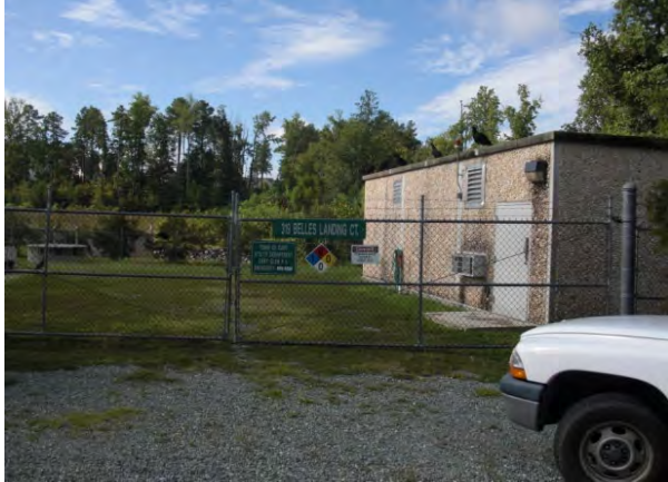
Cary Glen Pump Station
