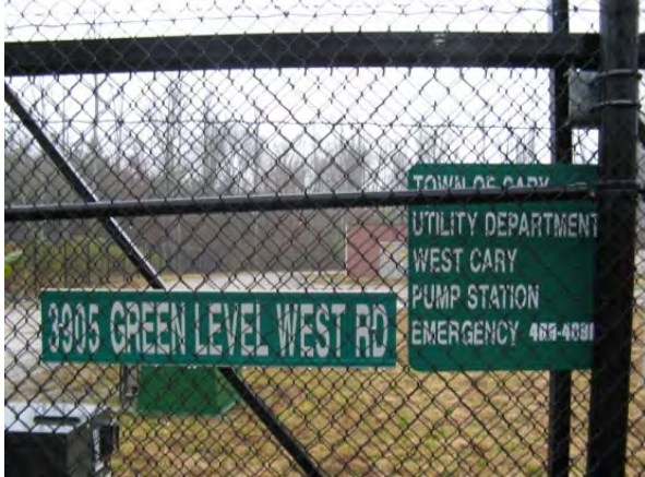
West Cary Pump Station
