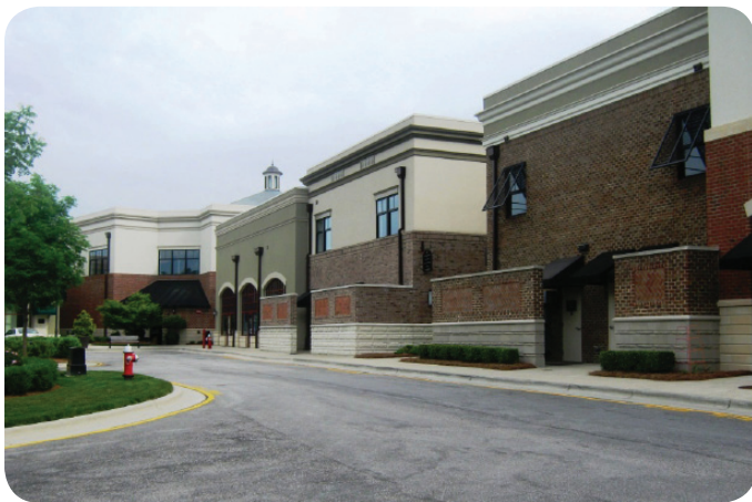
UTILITY AND LOADING AREA SCREENED BY MASONRY WALLS
