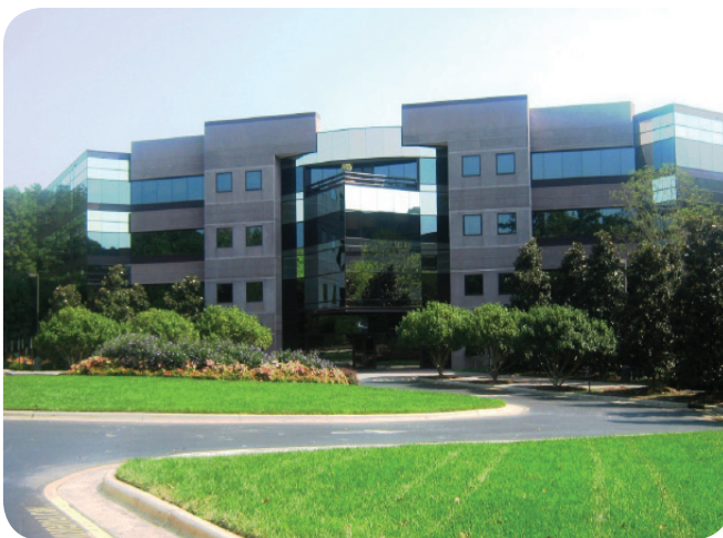
OFFICE BUILDING ENTRANCE LOCATED ON INTERNAL STREET
