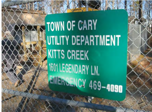
Kitts Creek Pump Station
