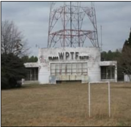
WPTF Transmitter Building, 833 East Chatham Street
