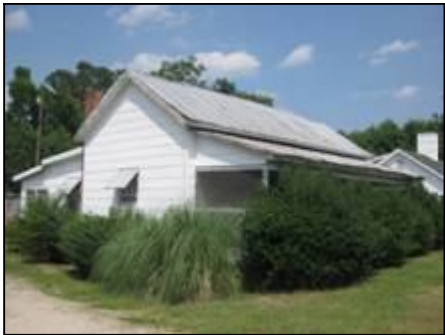
Byrd Tenant House, 0 Carpenter Fire Station Road
