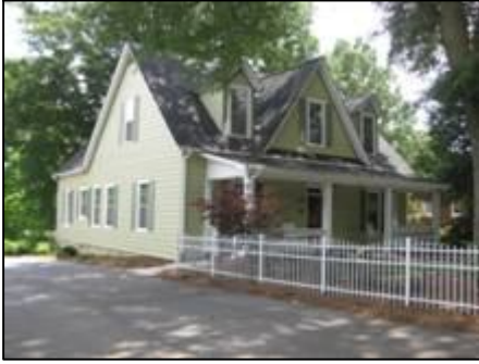
Pasmore House, 307 South Academy Street
