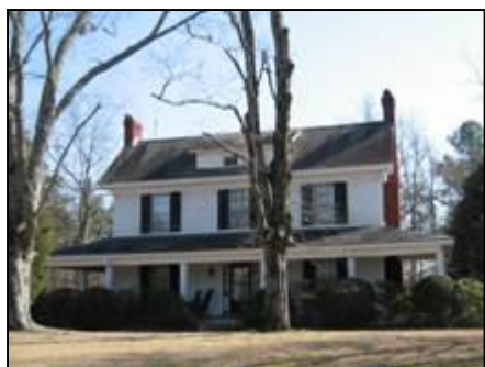
G.H. Baucom House, 2421 High House Road
