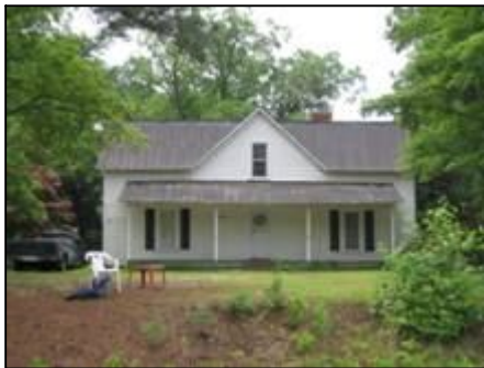
Buck Mills House, 3133 Green Level West Road
