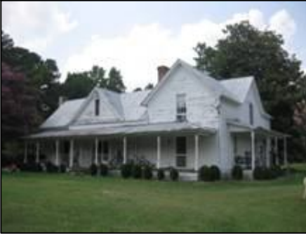
Yates-Carpenter House, 1116 White Oak Church Road
