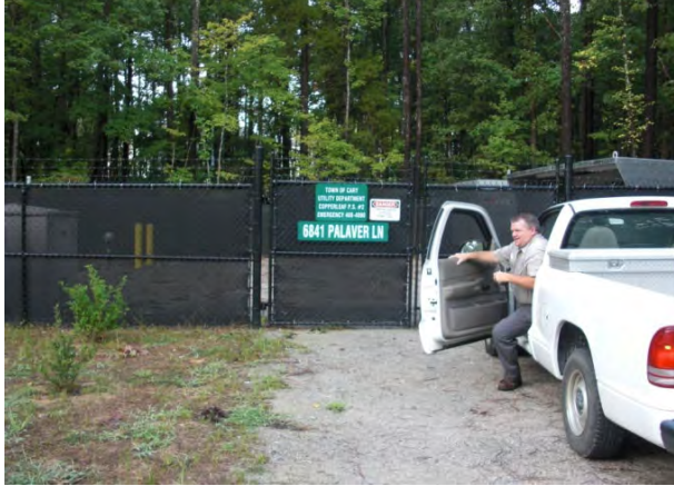
Palaver Pump Station
