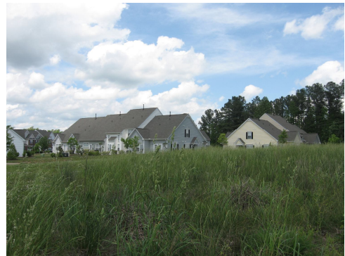
Fields that grew tobacco and corn now grow houses in many sections of Cary (North Woods Crossing Subdivision).
