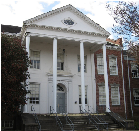
The former Cary High School building is being renovated as a community arts center.
