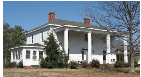
The Council House at 2420 Davis Drive is one of many historic properties inventoried in Cary.
