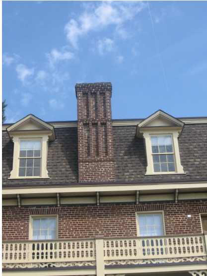
The roof features a chimney with distinctively detailed brick corbelling.
