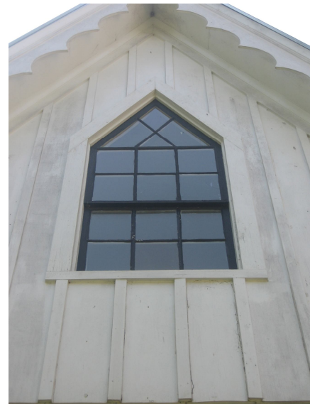
The dwelling has a board-and-batten exterior and characteristic Gothic arch windows.
